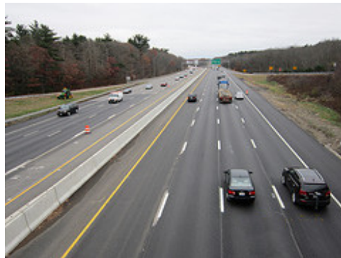
Numerous BMP's were required for the Add-A-Lane project to mitigate stormwater impacts from additional impervious area.
