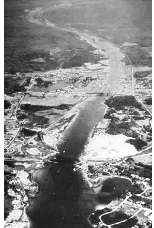
Early photograph of the Cape Cod Canal (Photograph courtesy of the US Army Corps of Engineers)
