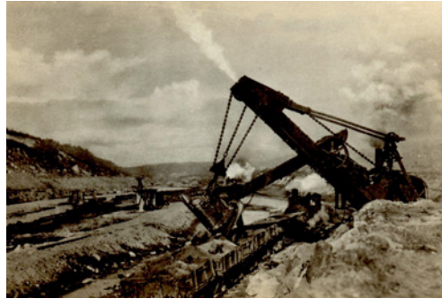
Digging the Cape Cod Canal. A steam shovel at work below sea level in the Collins Farm Cut
