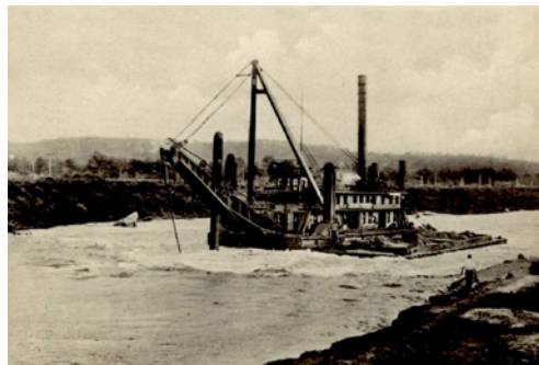
Dredge working in a strong current, July 1914 (Photographs courtesy of the Sandwich Glass Museum)
