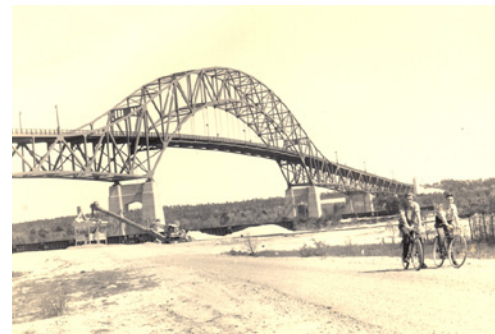
Sagamore Bridge under construction in 1934
