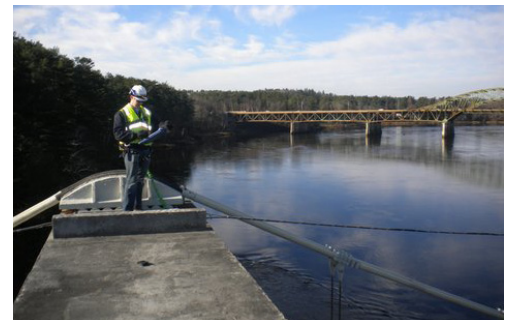
Rich Matson inspecting the Chain Bridge in Newburyport
